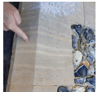
Ancaster Stone: a mid Jurassic limestone from Lincolnshire. Note "streaky bacon" appearance
