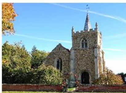
Colne church built mostly of sandstone cobbles and limestone, with some flint
